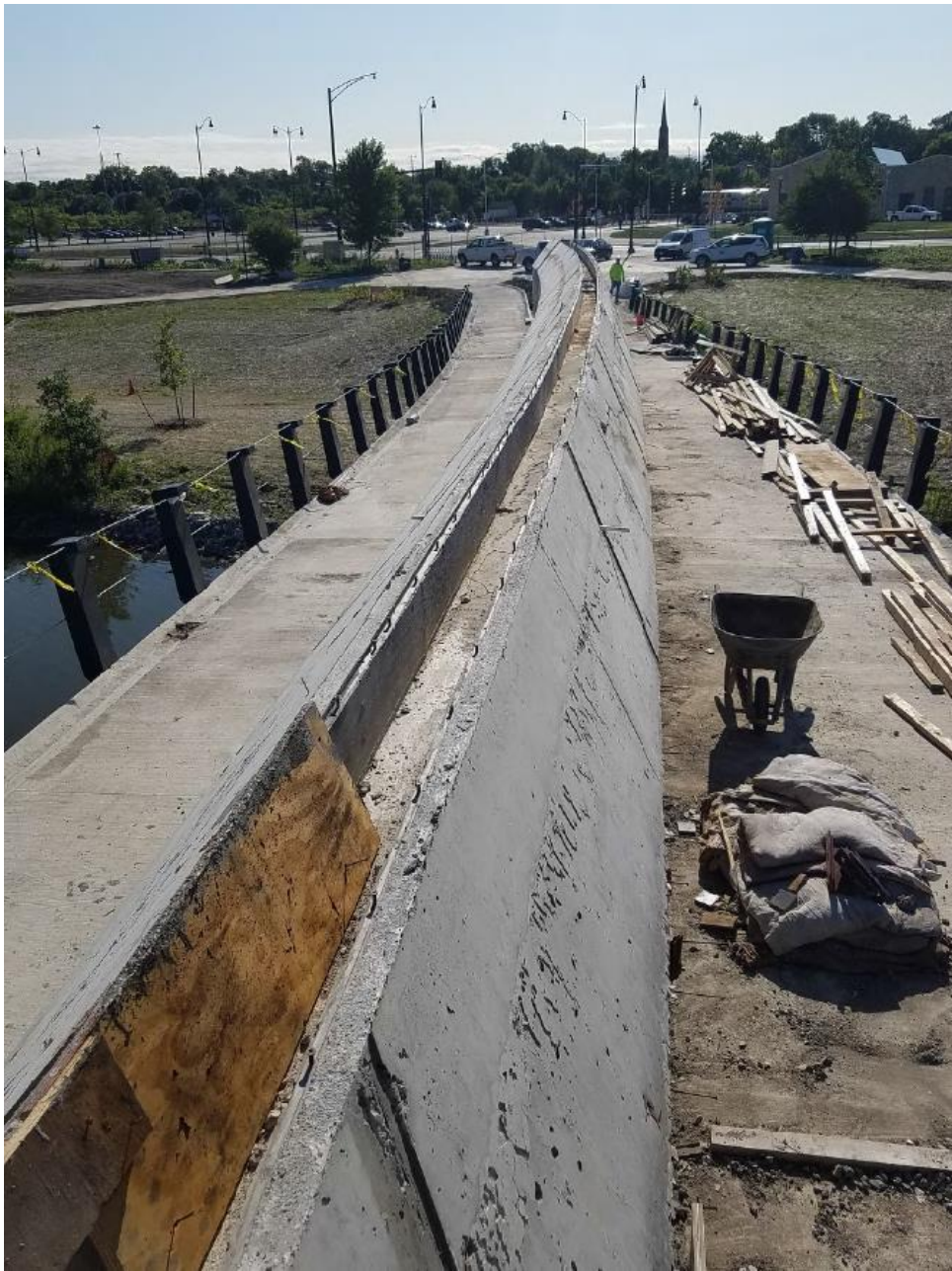
August 4, 2020. Top section of cornice, pour concrete channel for cornice lighting. Looking east.
