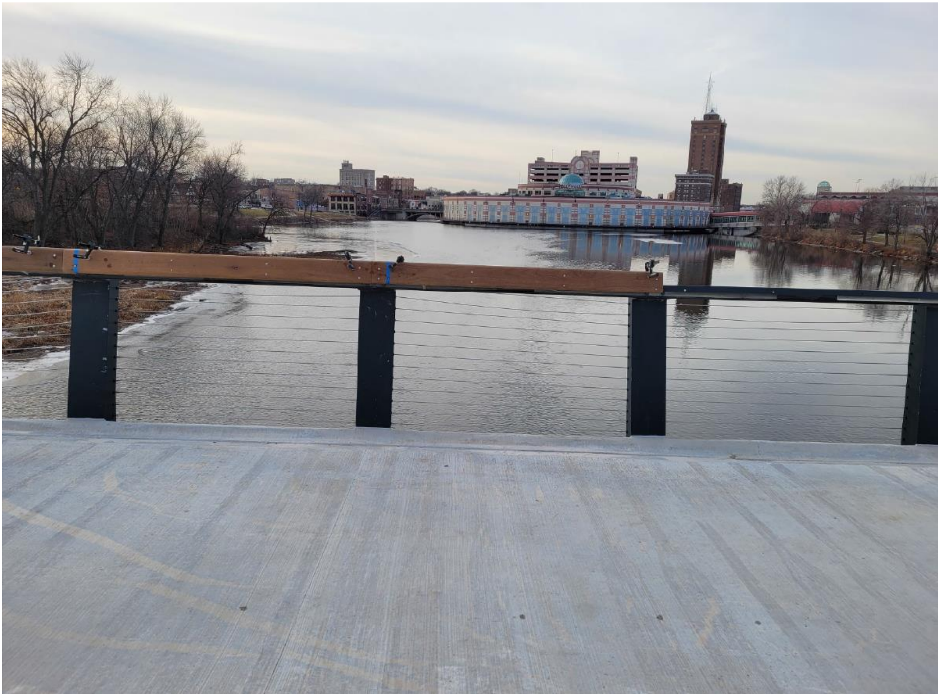
12/15/2020- Bridge view-Looking south.
