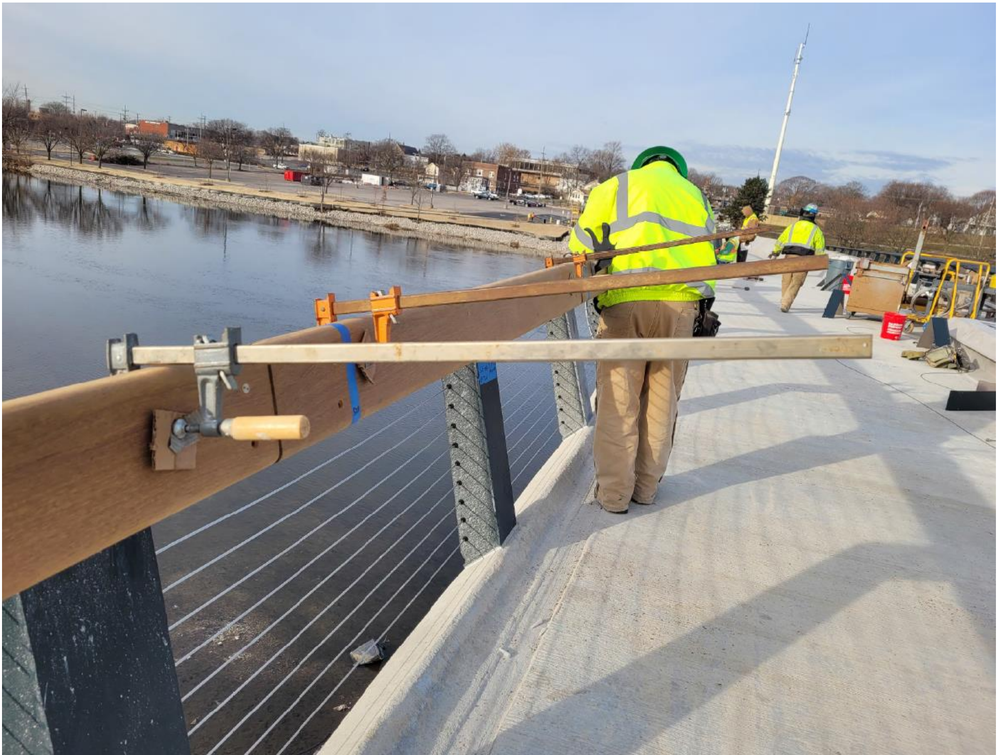
12/15/2020- installing IPE handrails and adjusting steel cables.
