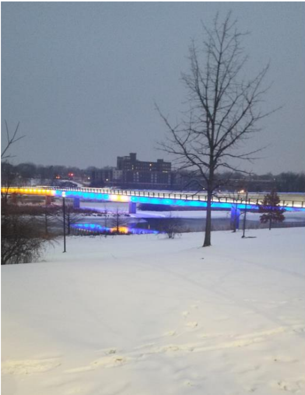
01/06/2020- Bridge View. Looking west. Under bridge lighting test.
