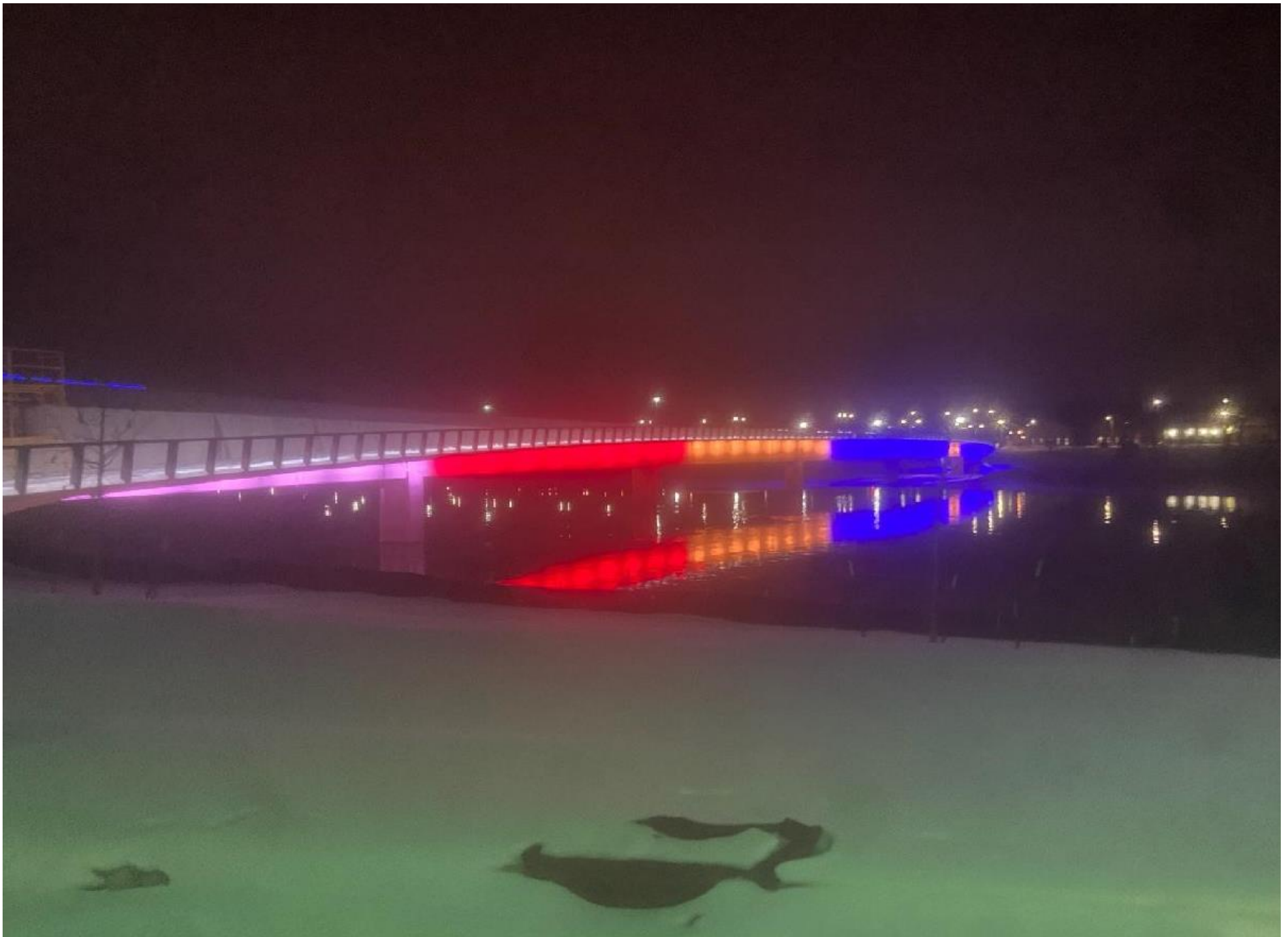
01/07/2021-Under bridge lighting test. Looking NE
