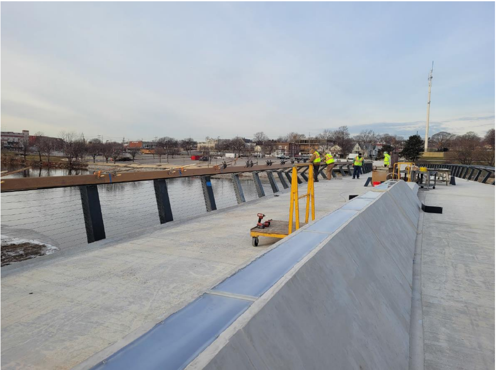
12/15/2020- installing IPE handrails and adjusting steel cables.
