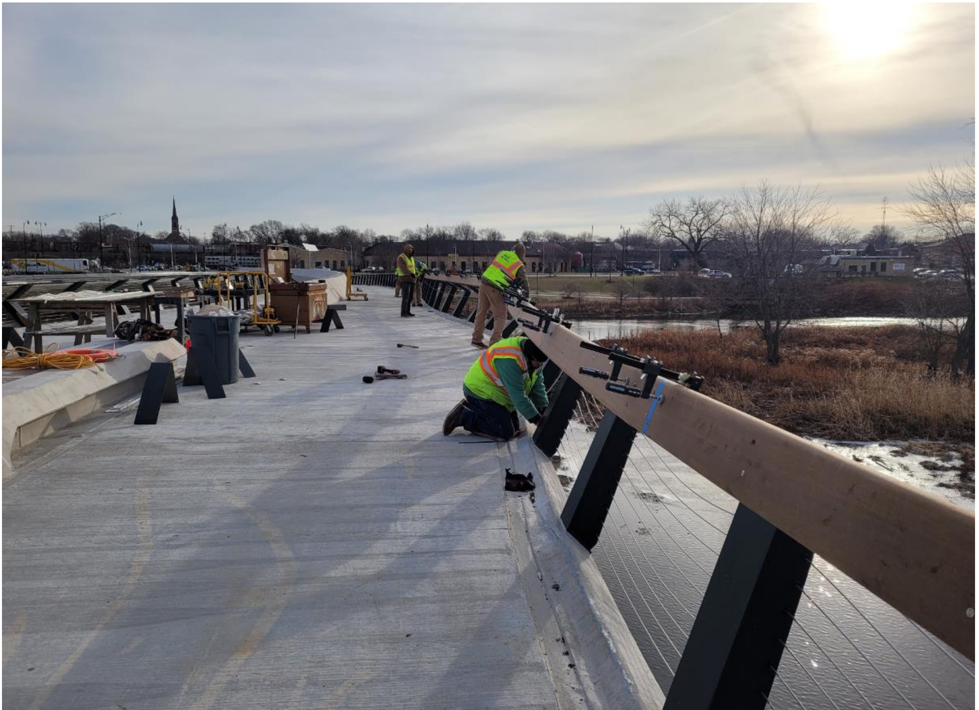
12/15/2020- installing IPE handrails and bridge rail lightings.
