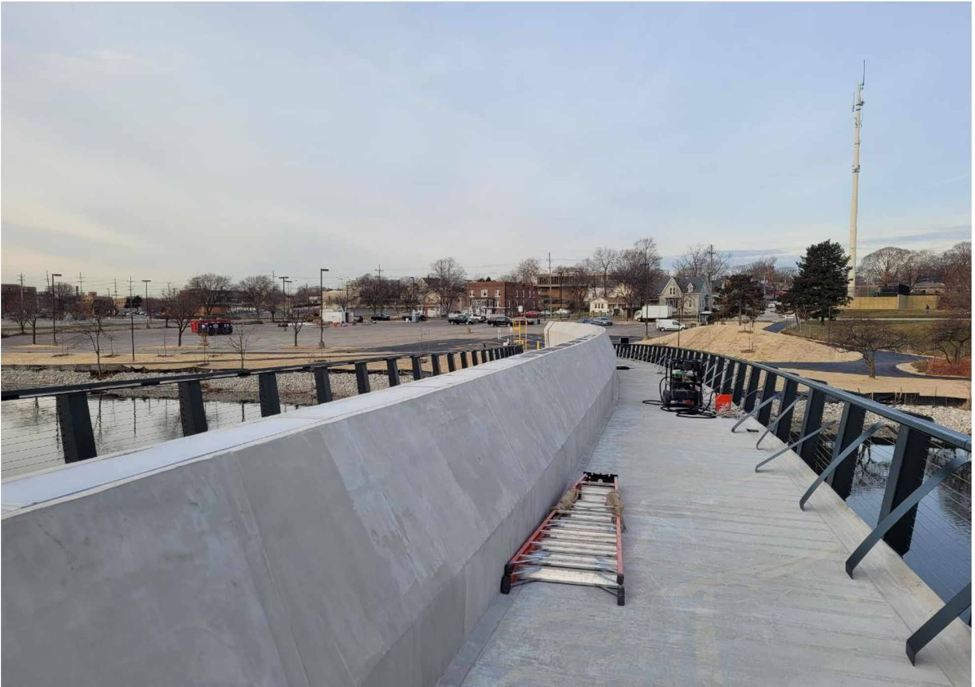
12/15/2020- Bridge view- Looking west.
