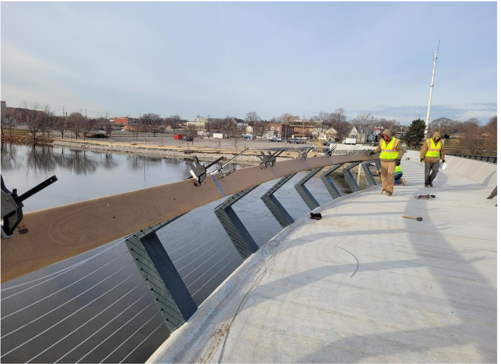
12/15/2020- installing IPE handrails and adjusting steel cables.
