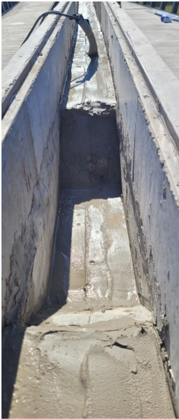
05/12/2021-Continue cornice channel work, sloping channel to drain to drain pipe. Span 5-7
