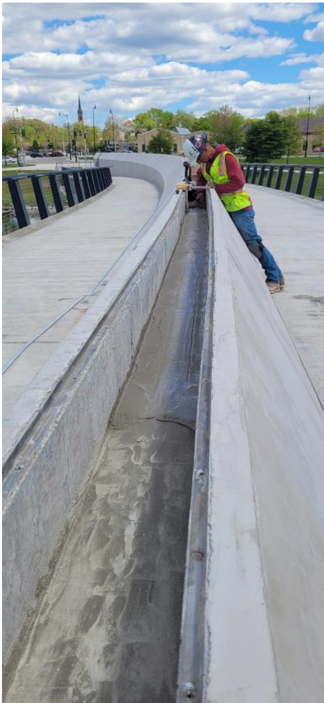
05/14/2021-Contractors continue cornice channel work. Span 5-7
