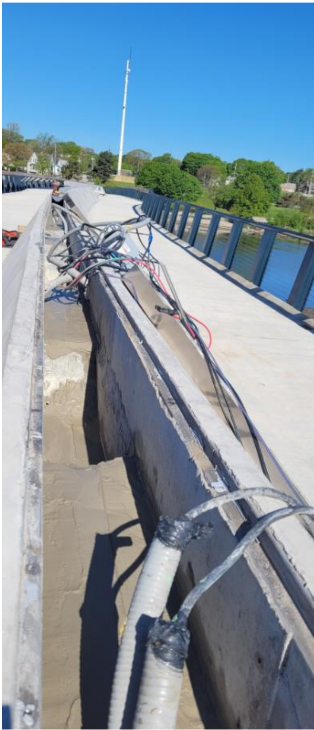
05/12/2021-Continue cornice channel work, sloping channel to drain to drain pipe. Span 5-7
