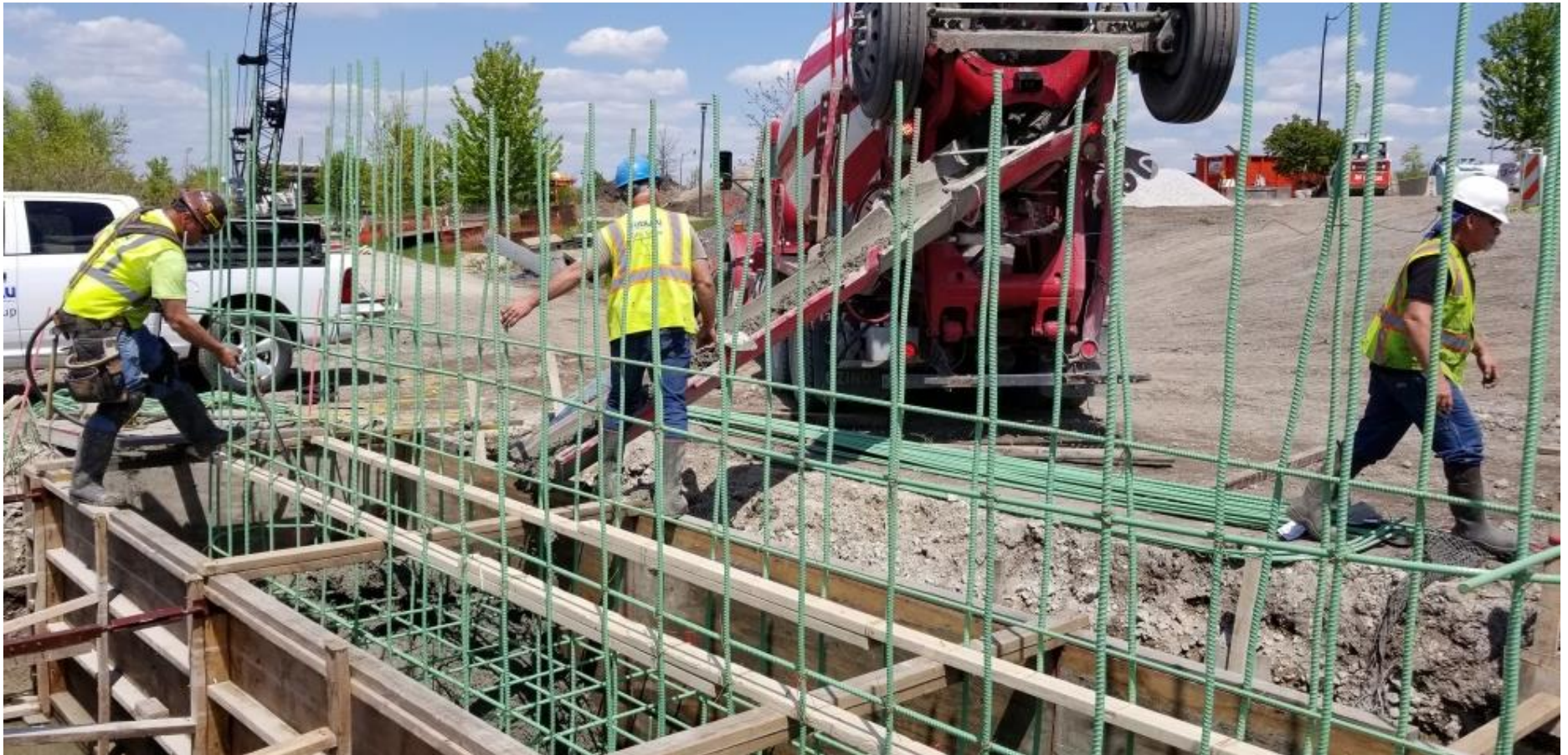
Pouring concrete- east abutment footing 05/14/2019
