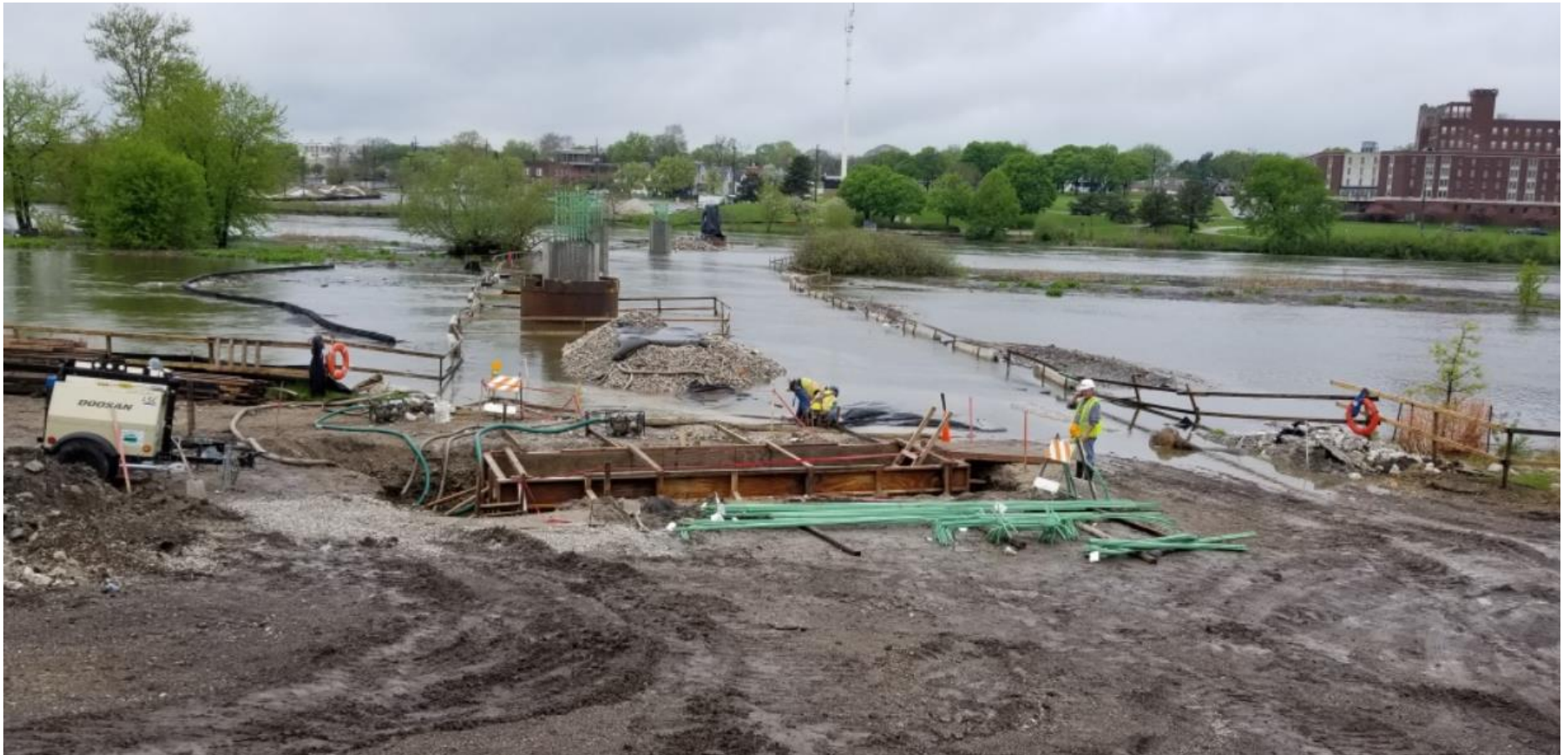
East Abutment work-forming abutment footing – River at flood stage- 05/09/2019.
