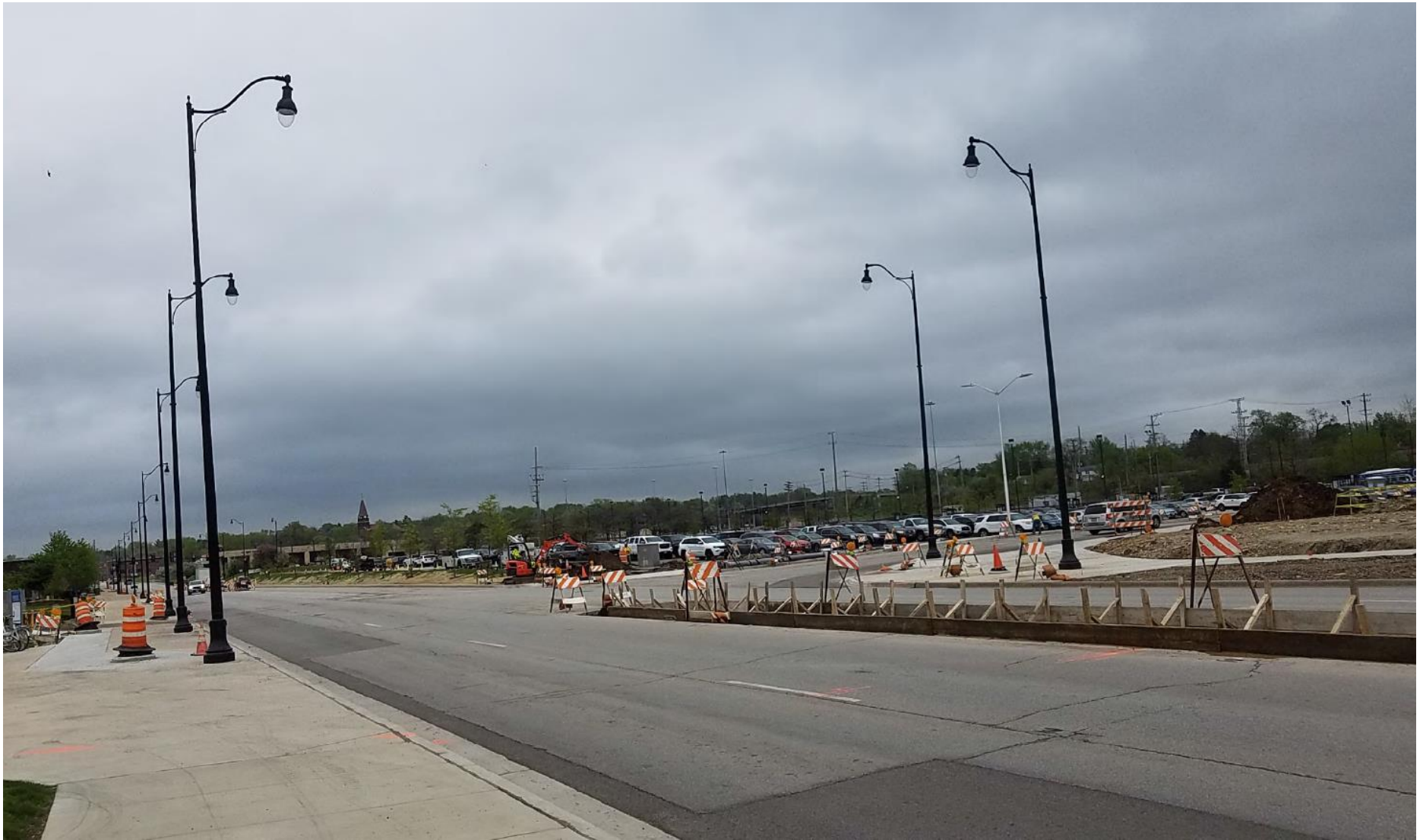
Stage 5- Median work along Broadway Avenue. Median graded and curbs formed. Ready for pouring concrete and backfilling.
