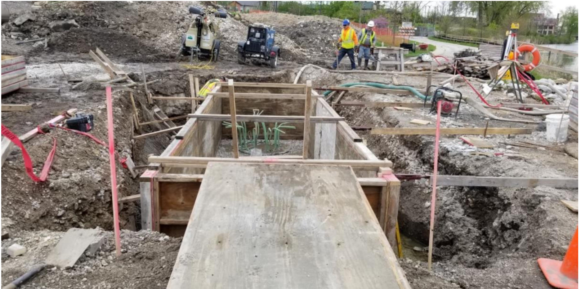
East Abutment work-forming abutment footing - 05/08/2019.
