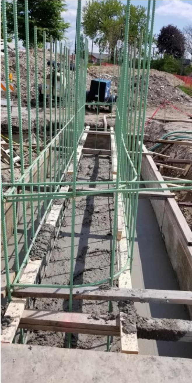
Pouring concrete- east abutment footing 05/14/2019
