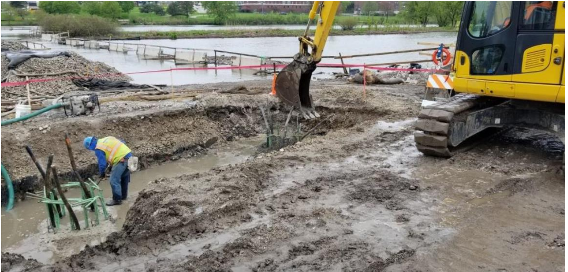
East Abutment work- forming/excavation of abutment footing - 05/07/2019.
