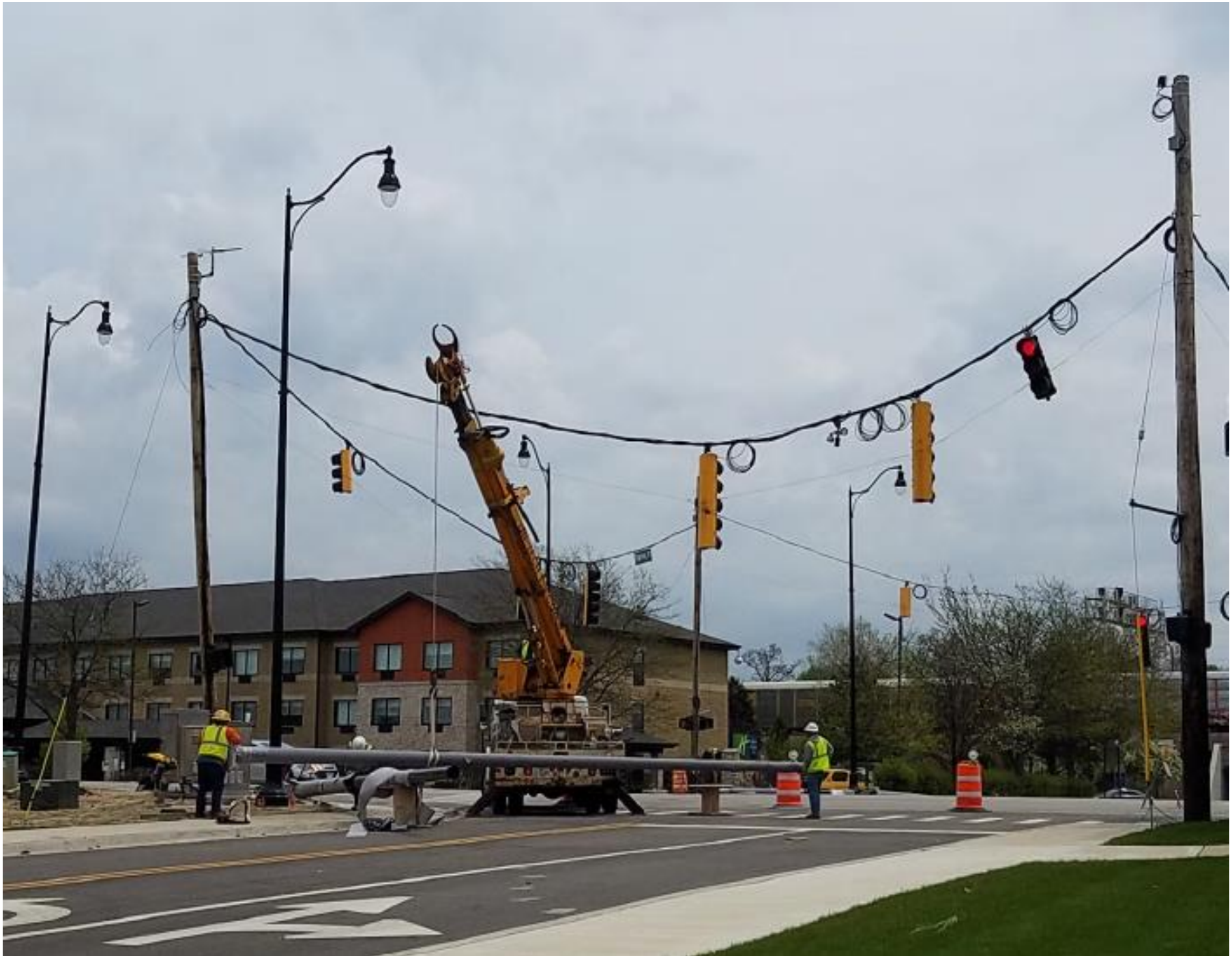
Stage 4- Traffic signal at Broadway Avenue and Spring Street being install.
