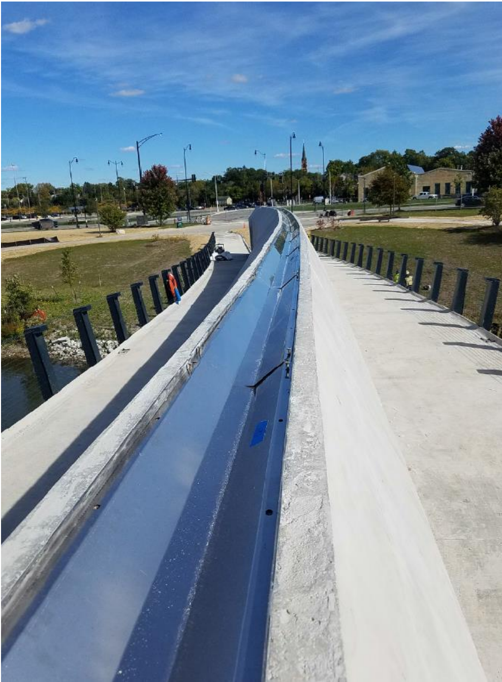
Installation of cornice metal channel for upper box lighting. 10/2/2020
