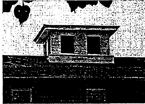
Cupola on the main house. Cupolas helped facilitate airflow, and were not merely decorative.
