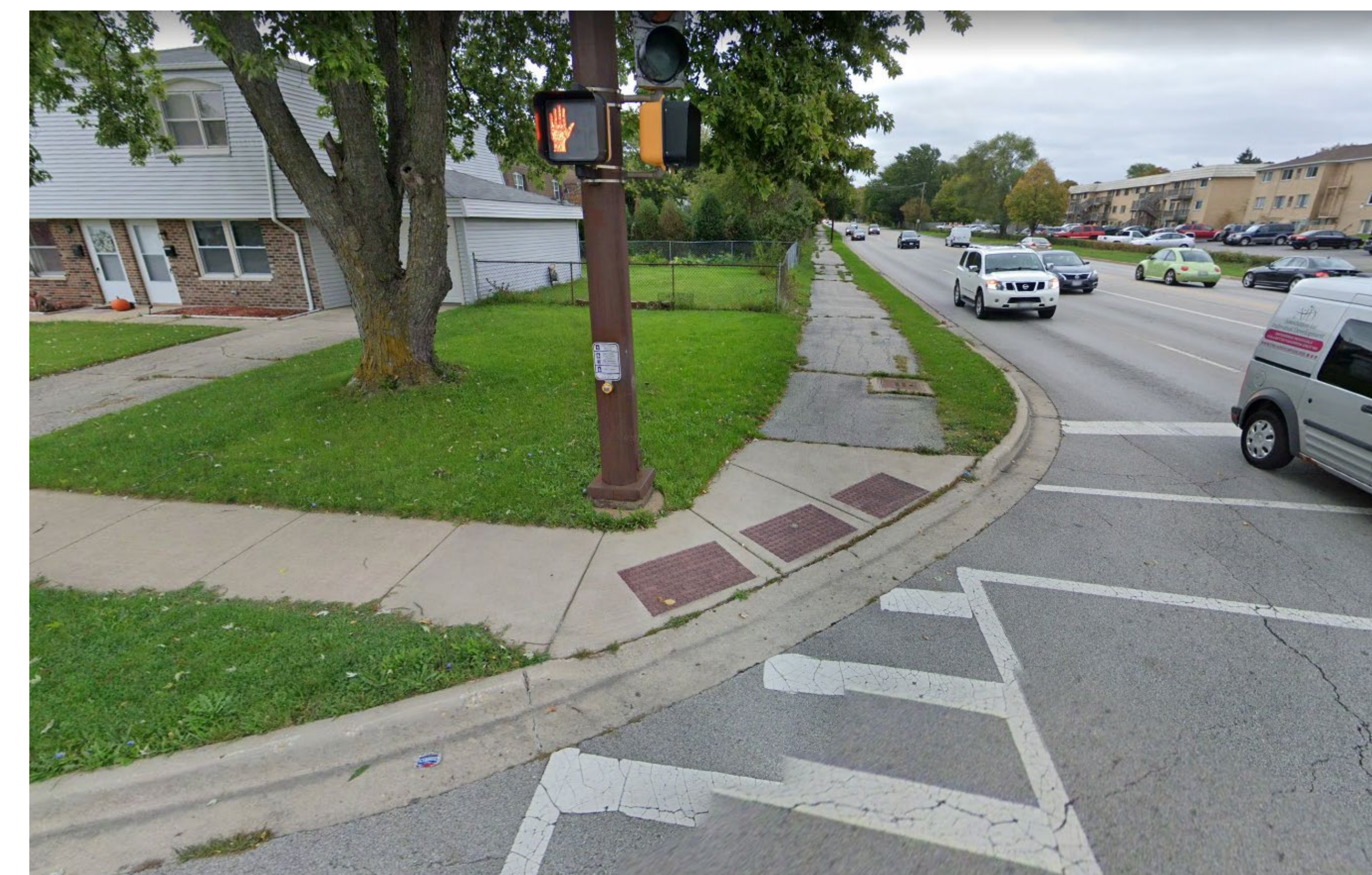
Noncompliant ADA sidewalk
