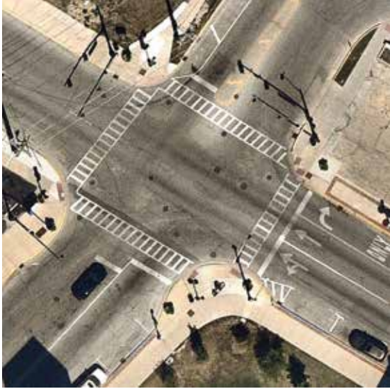
EXISTING INTERSECTION (W. NEW YORK/RIVER)
