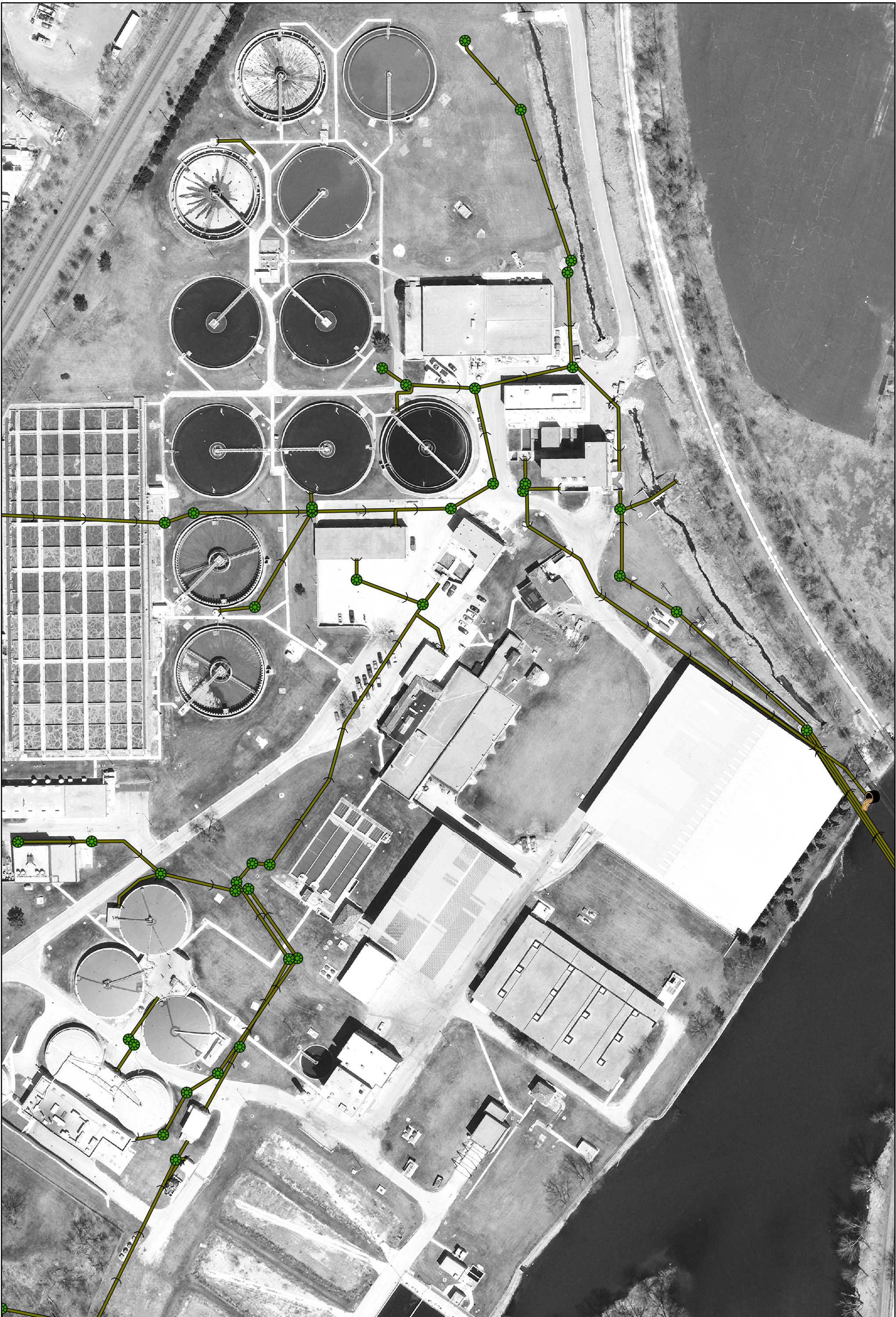
Figure 18 Fox Metro CSO - 002 Fox Metro Plant
