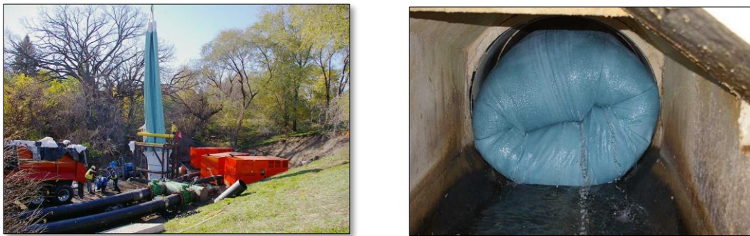
Figure 18: Cured-in-Place Pipe Liner Installation
