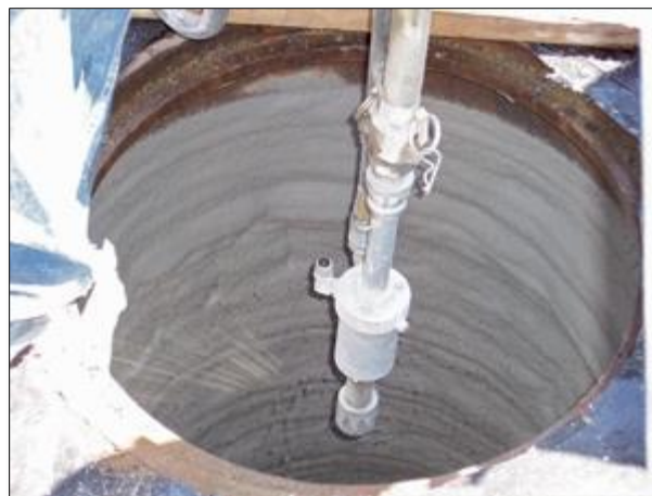
Figure 19: Monolithic Cementitious Manhole Liner
