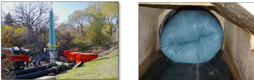
Figure 18: Cured-in-Place Pipe Liner Installation
